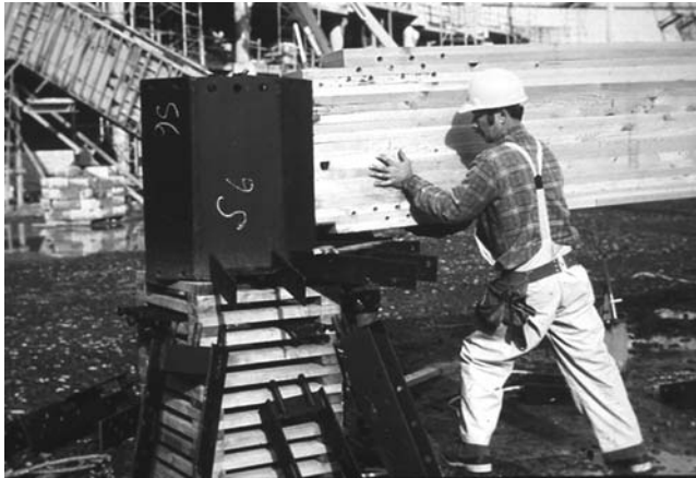
FIGURE 10.3 Large composite beam made from laminated lumber.
