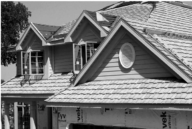
FIGURE 13.7 Wood fiber plastic roofing tiles.
