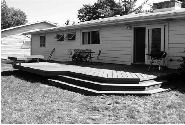
FIGURE 13.6 Wood fiber plastic deck.
